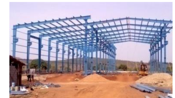
Pre Engineering Building
