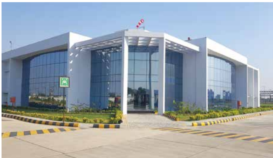
► Manufacturing facility at Goindwal, Punjab
