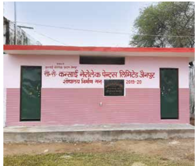
► Construction of toilet in school
