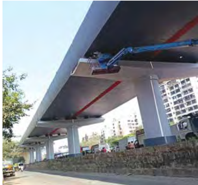
▲ Anticarbonation Paint Application
