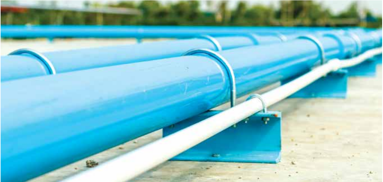
▲ Pipe Coating Application
